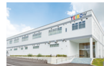
MIM Development Center (Miyakoda-cho, Kita-ku, Hamamatsu City)
